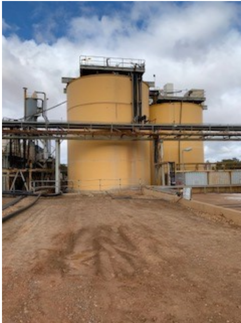
Exhibit 16 – Wonawinta Plant – Fully Refurbished - Leach Tanks, New Larger Ball Mill, New Diesel Generators
