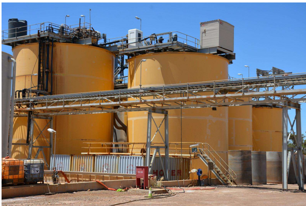
(Figure 6 - Refurbished leach tanks at Wonawinta plant)
