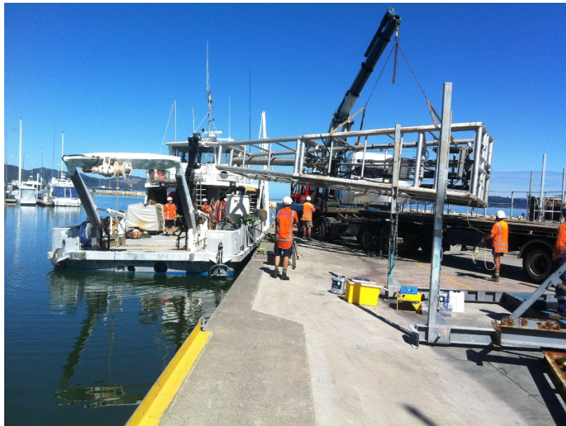
Figure 26 Mobilisation of the Deep Drill Rig
