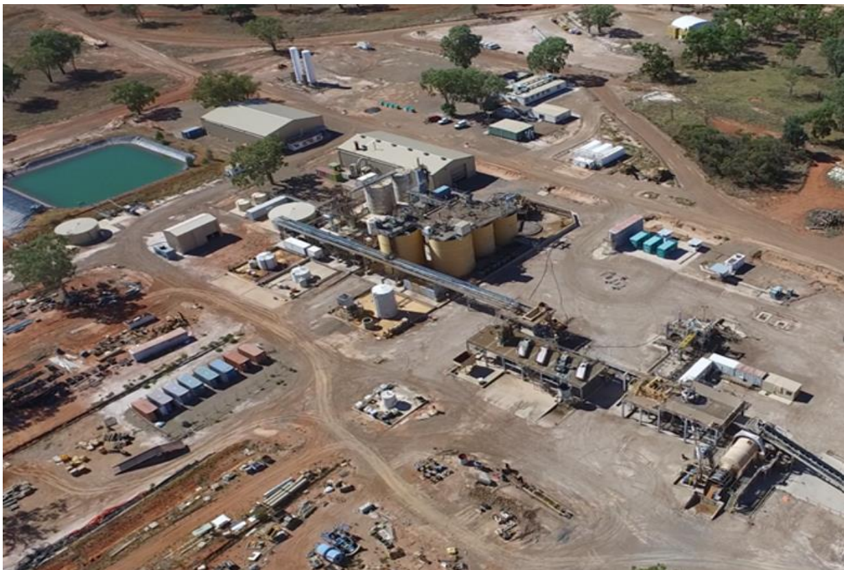
Figure 4: The existing Wonawinta CIL Processing Plant
